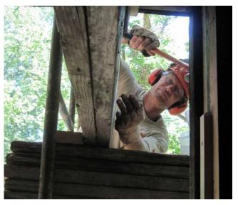
*"The Log Whisperer"* pounds in braces to support cabin to remove & replace 3 logs, repairing several others.
